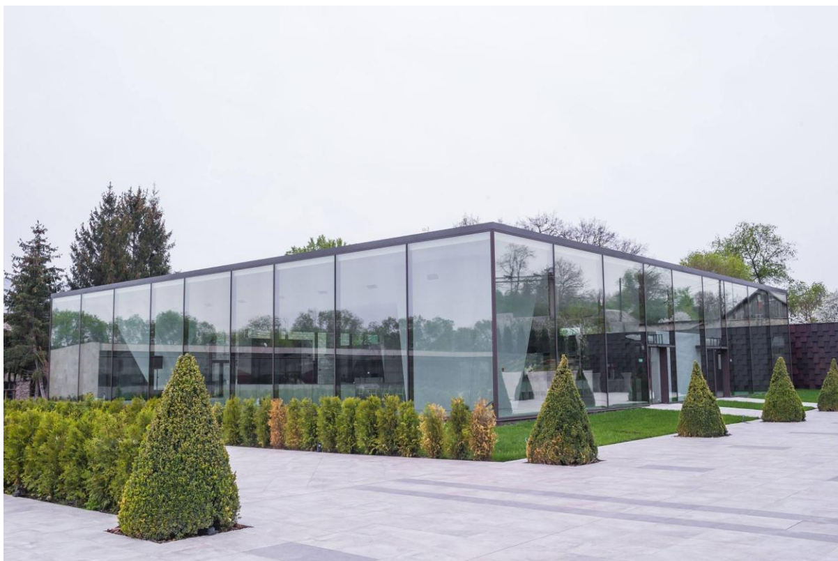
Figura A4.5. Pavilion multifuncțional ( https://castelmimi.md ; accesat 28.05.2019)
